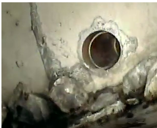
Figure 3-4: 200mm dia. PVC Outfall Pipe Inside the Garage Culvert
