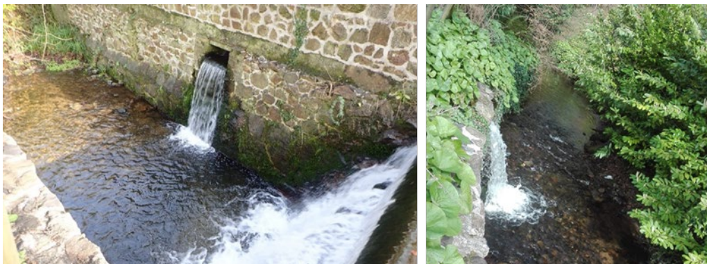
Figure 3-1: Surfacewater Outfalls Downstream of the Weir/Drop Structure
