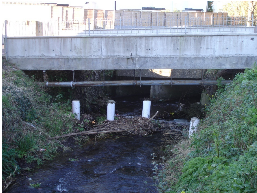
Figure 3-16: 150mm dia. Water Main Upstream of the Twin Culvert
